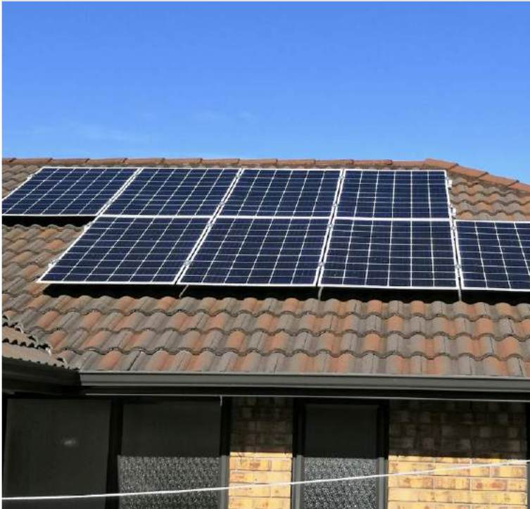
The McNae's 5kW System in Auckland "The biggest benefits is that it heats our hot tub"
