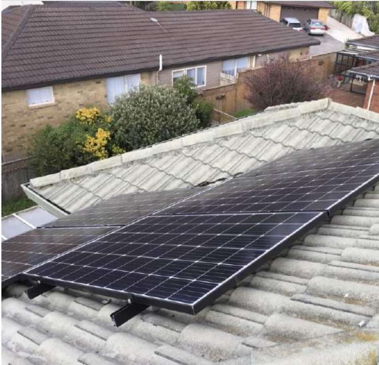
The Yates' 2.7kW System in Auckland "It's nice to have some of our power for free"
